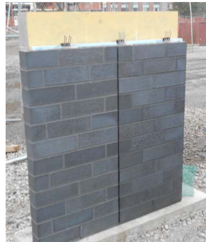
Figure 4: Typical Wall mock-up Photo by SKANSKA Inc.
