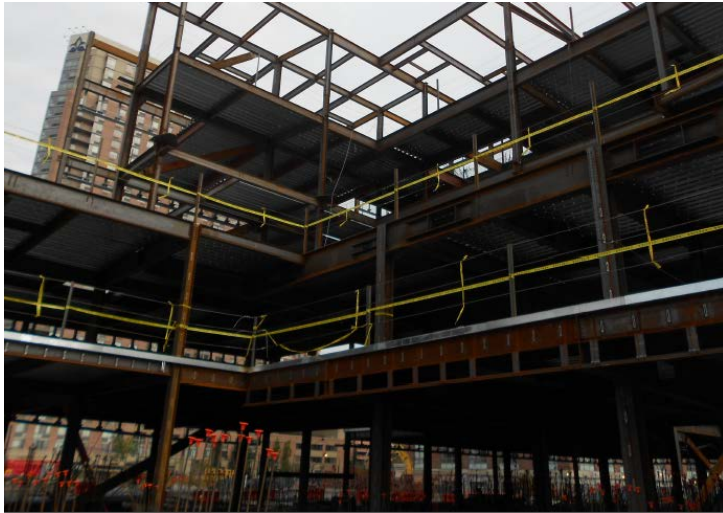
Figure 14: Steel Frame Erection Photo by SKANSKA Inc.
