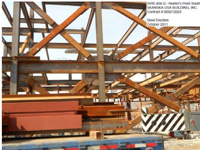
Figure 17: Lateral bracing erected
