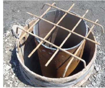
Figure 9: Isolation Casing Photo by SKANSKA Inc.
